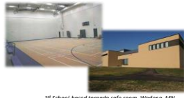
1 st School-based tornado safe room, Wadena, MN (2012) following June 17, 2010 tornado damage
