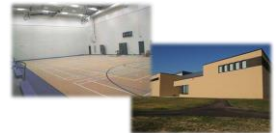
1 st School-based tornado safe room, Wadena, MN (2012) following June 17, 2010 tornado damage
