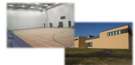
1 st School-based tornado safe room, Wadena, MN (2012) following June 17, 2010 tornado damage
